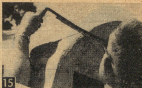
15 Rounding off corners of roof and side wall with drawknife.
